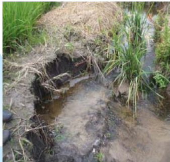
*1 Levee collapsed due to water erosion
