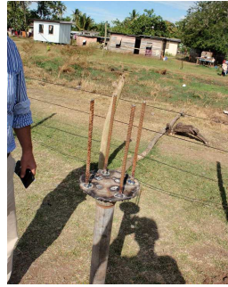
Details of iron frame used at Fiji
