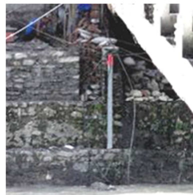
Installation on a revetment (Nepal 2010)
