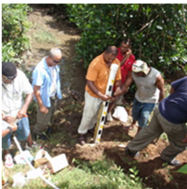
Installation on iron angle pile (Fiji 2011)
