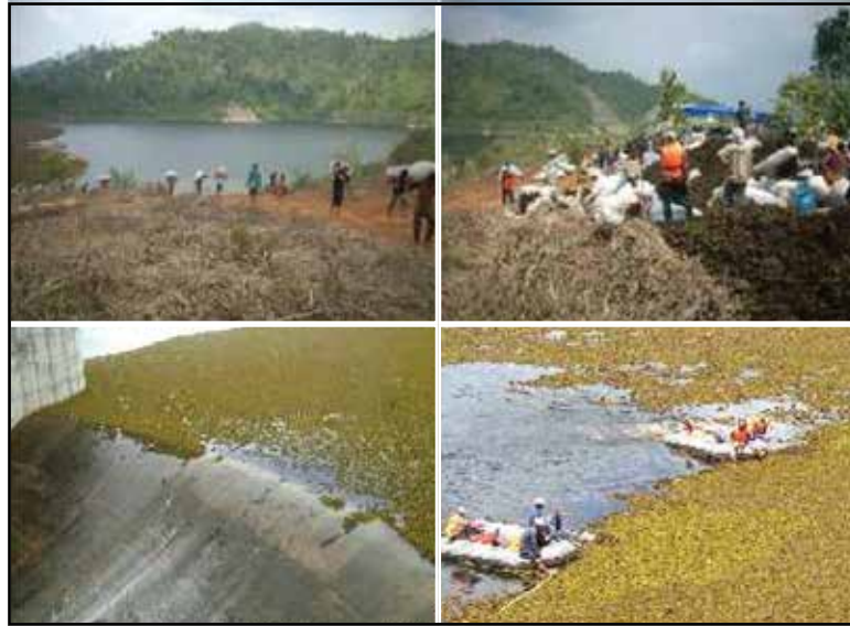
Figure 10: Over flow in Batutegi Reservoir Spillway
