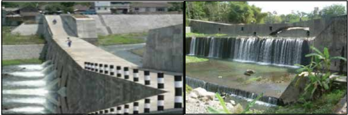
Figure 26: Tulungrejo Check Dam and Jambe Wangi Sabo Dam
