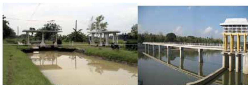
Figure 20: Sempor Main Canal and Sapon Weir
