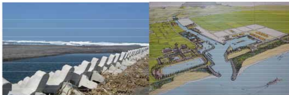
Figure 25: Wave Breaker at Glagah Beach and Its Development Plan
