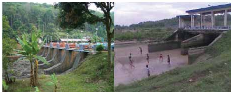
Figure 11: Jelok Weir and Klambu Weir
