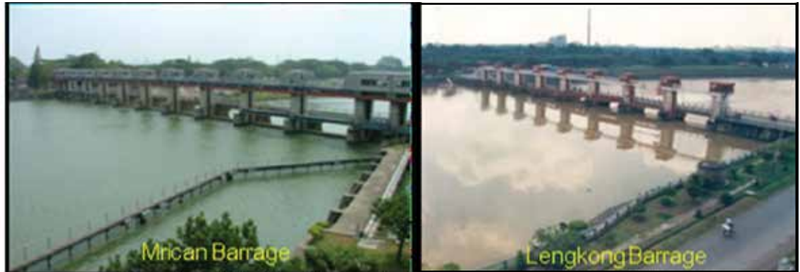
Figure 14: GerakMrican Weir and Lengkong Weir
