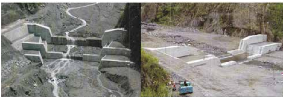
Figure 14: Sabo Dam 7-5 and 7-7 Source: Hazama Co.
