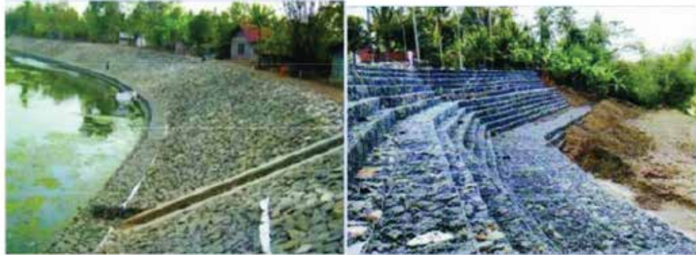
Figure 23: Revetment of Luk Ulo River
