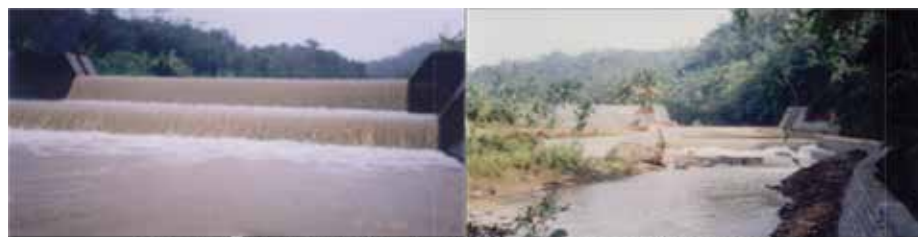
Figure 16: Goler Check-Dam and Pisitan Check-dam
