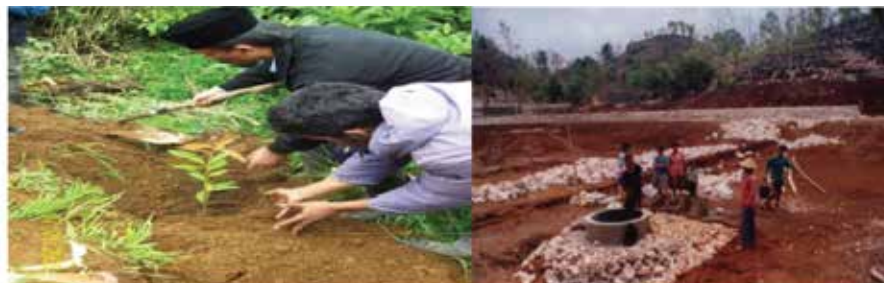
Figure 18: Trees Planting and Construction of Infiltration Wells
