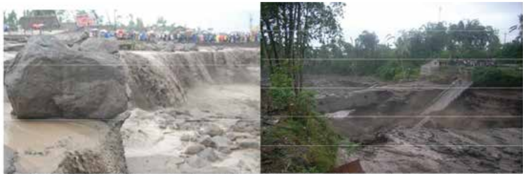
Figure 11: Debris Flow and the Collapse of Tlatar Bridge
