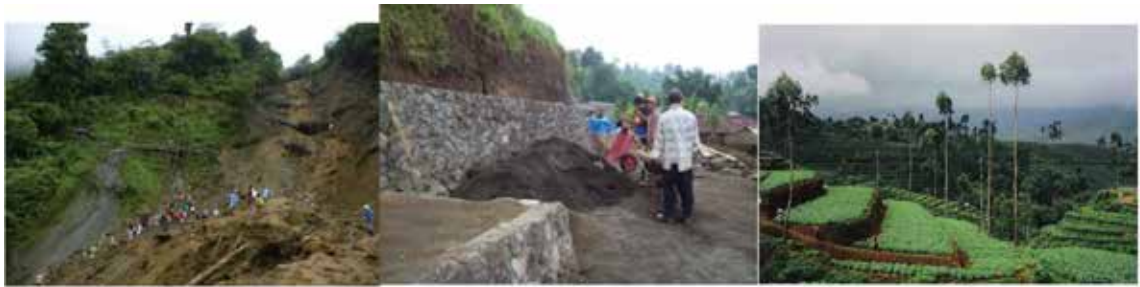
Figure 20: Landslide Management by Vegetative, Structural, and Non-Structural Methods
