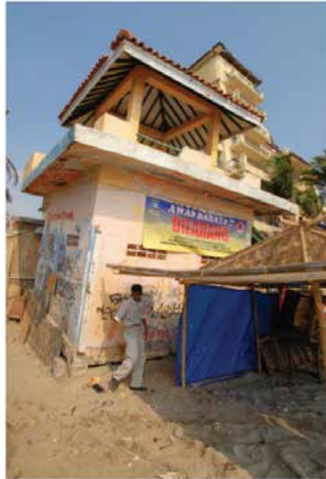
Figure 9: Abraded SAR Post
