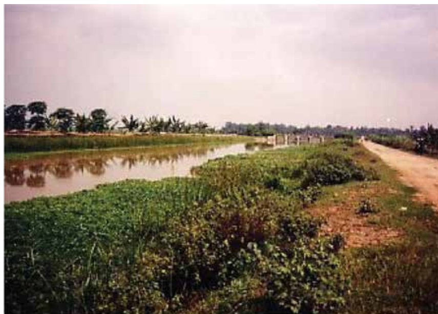
Figure 5: Channel Narrowing in Sindupraja Main Canal, Majalengka Regency
