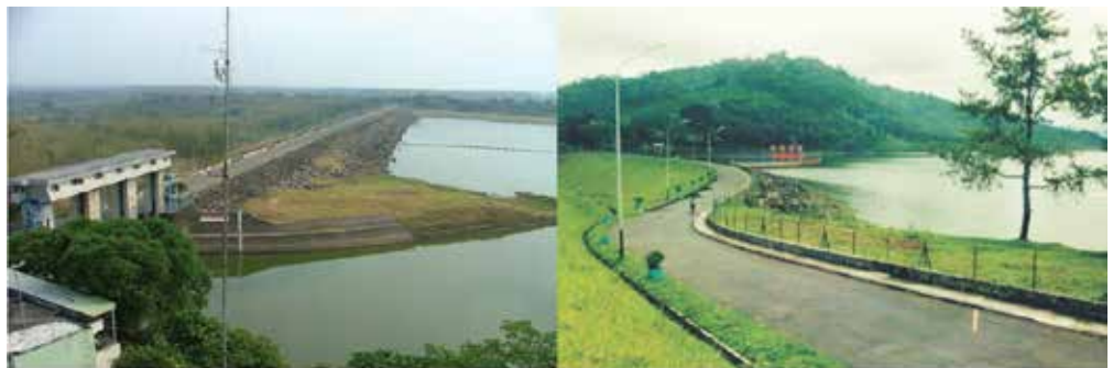
Figure 10: Wonorejo Dam and Selorejo Dam
