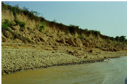
Photo 7 Cobbles on the eroded riverbank (February 1998)
