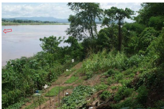
Photo 8 No. 1 groyne concealed by vegetation (June 2010)
