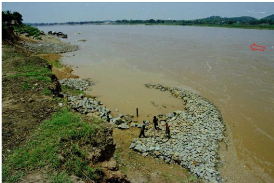
Photo 5 No.1 and 2 masonry under construction (May 1998)
