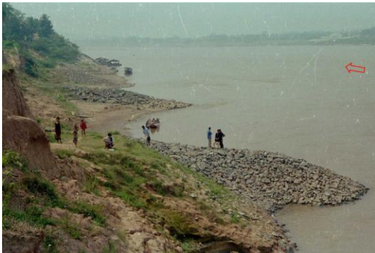
Photo 6 No.1, 2, 3 and 4 masonry completed (April 2000)
