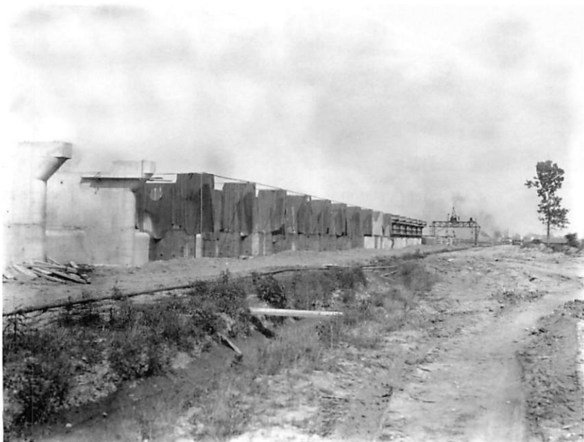
High strength concrete used in the spillway was an engineering advancement.
