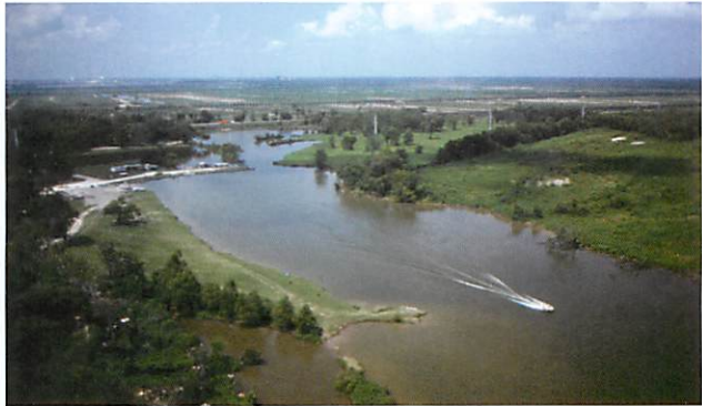
The largest developed recreation site in the spillway is located along the lower guide levee adjacent to Highway 61.
