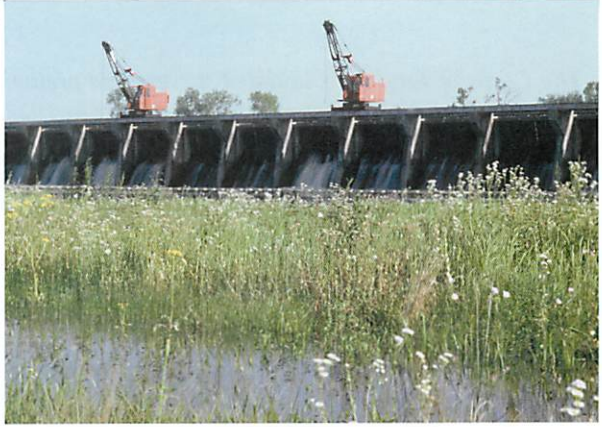
Wildflowers enliven the lakeside of the structure during spring high water.
