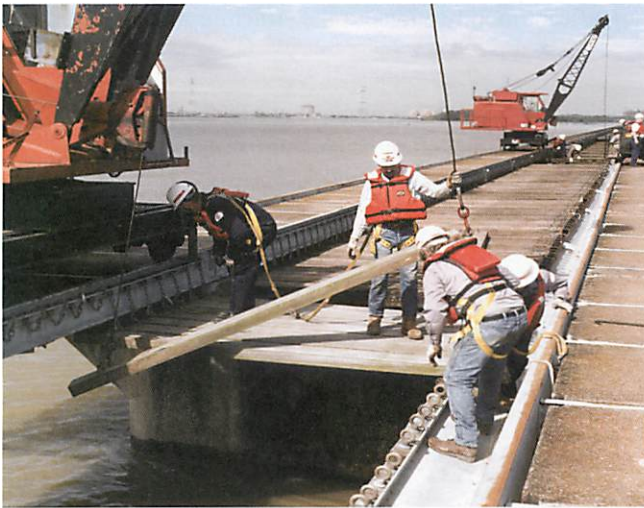
In opening the spillway, each timber is individually lifted and placed atop the structure.
