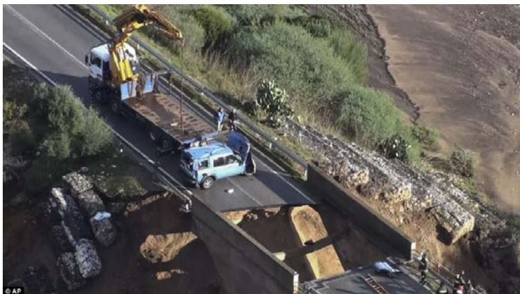
This picture, issued by the Italian Police, shows a wrecked police car recovered from a crack in a bridge that was caused by torrential rains, in Dorgali, Sardinia
