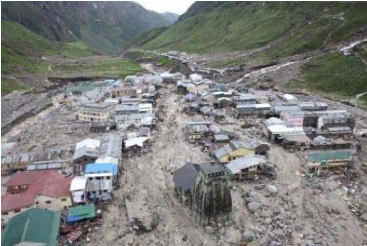
The Kedarnath Temple (C, foreground) amid flood destruction in the holy Hindu town of Kedarnath, located in Rudraprayag district in the northern Indian state of Uttarakhand, on June 18, 2013. (STRDEL/AFP/Getty Images)
