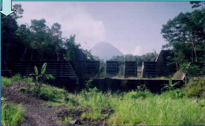
BO-D5, Slit Type Check dam
