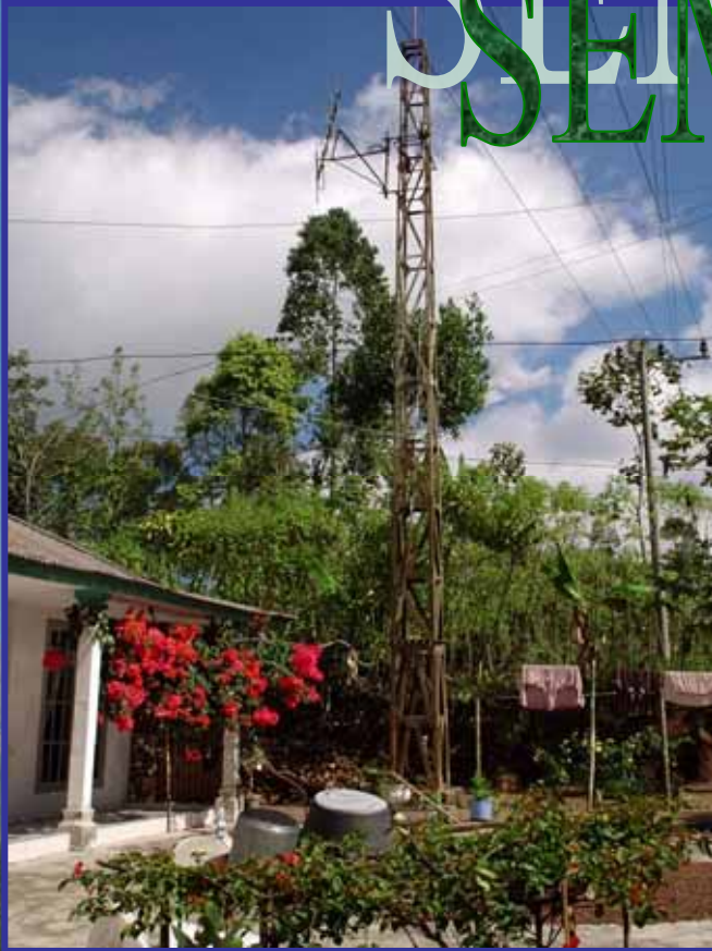
Station of Lahars Warning System in Lumajang
