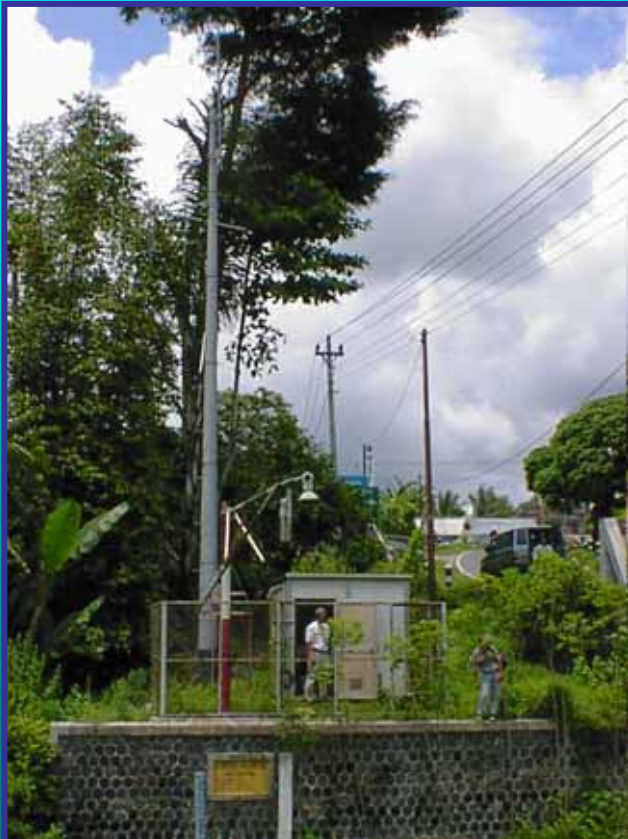
Automatic Water Level Gauge in Pulowatu
