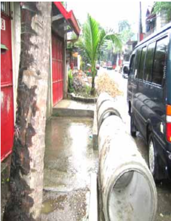
IMPROVING THE DRAINAGE SYSTEM BY PUTTING BIGGER SIZE OF CULVERT
