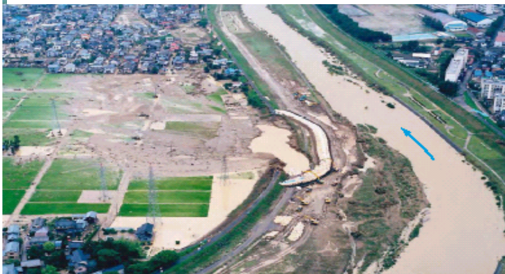
Restoration work from disaster
