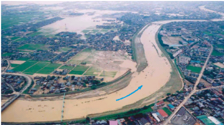
Broken point of the embankment
