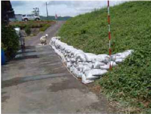
Shimizuchou, Katakasu : water leakage at the left bank of Hino River
