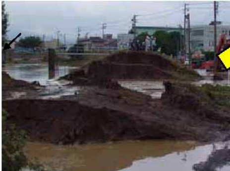
Dyke breaks ( Asuwa River in Fukui district)
